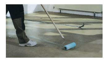
• Primer is used before self-leveling cement, to close the pore and crack on subfloor, reduce the absorptive character, at the same time, it can increase the adhesive ability between subfloor and adhesive.
